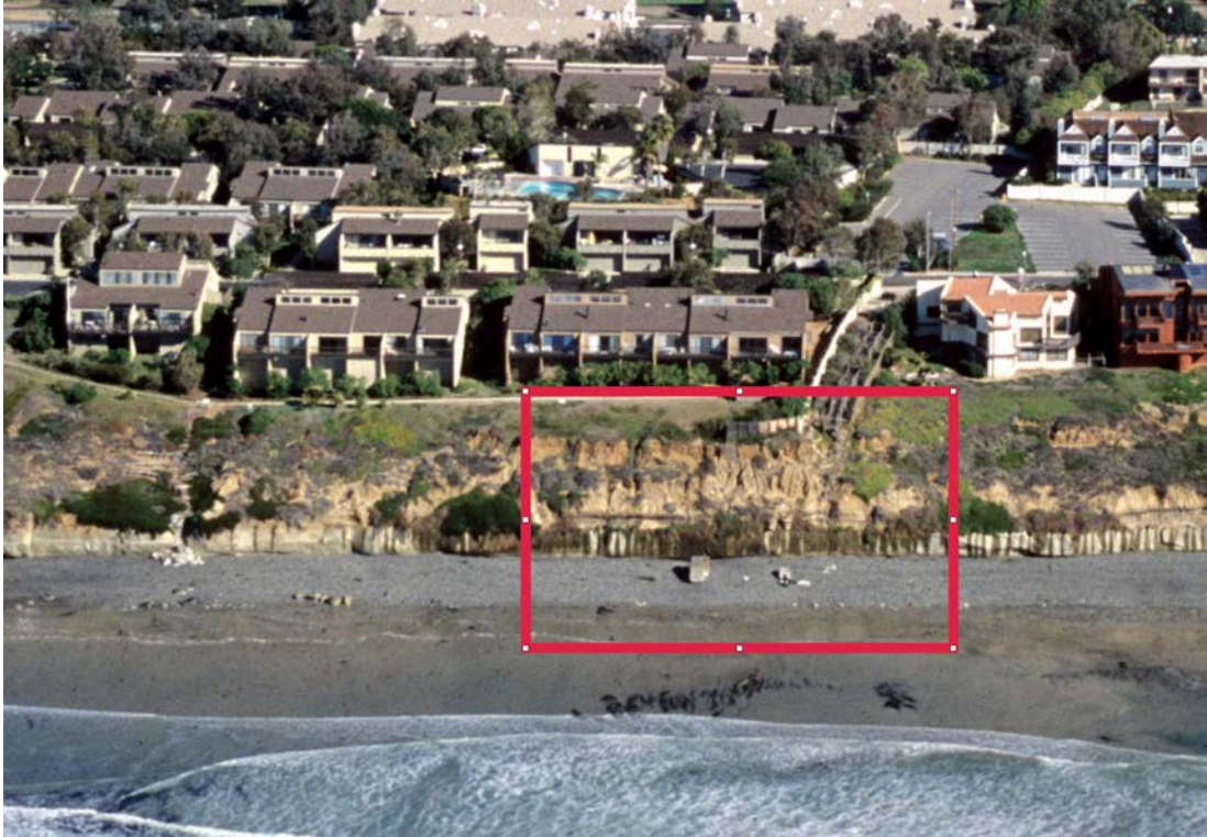
January 1989: Before rebuilt stairway
